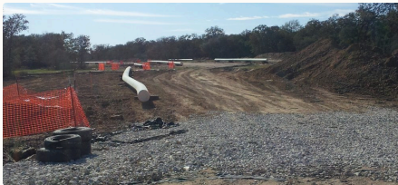
Illustrative: pipeline. Photo: KenB, CC BY-SA 3.0
